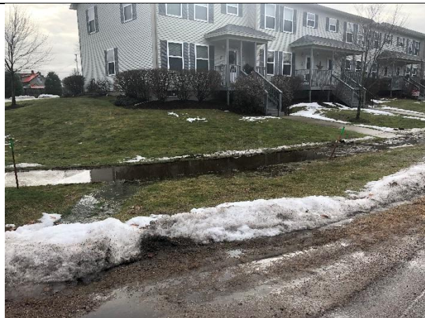
Photo 2: Runoff ponding on sidewalk along Checkerberry.
