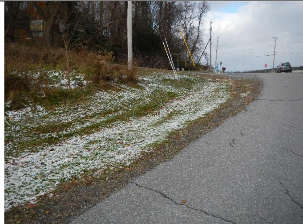
Photo 1: Sharp bend at bottom of Crest Dr, runoff flows on to Howard Dr Photo 2: Grassed ditch along Howard Drive
