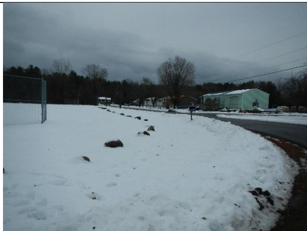
Photo 1: Grassed swale along Bradley Ave with a low point on bend.
