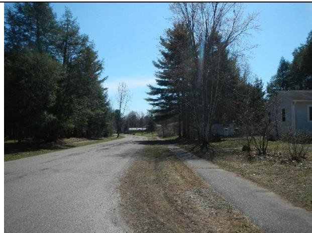
Photo 2: Gravel and grass shoulder along the west side of Kingswood Drive provides some room for stormwater treatment.
