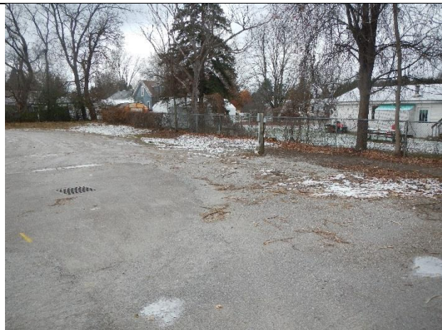
Photo 2: Dry well in unpaved portion of parking lot
