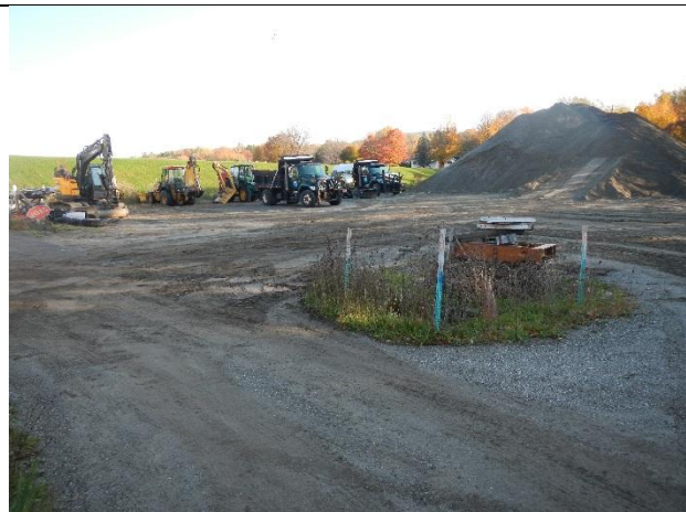
Photo 1: Large gravel/dirt area draining to catch basin
