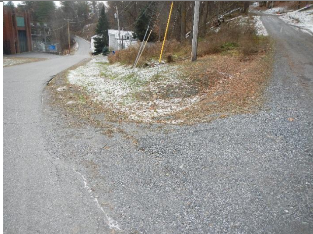
Photo 1: Sharp bend at bottom of Crest Dr, runoff flows on to Howard Dr Photo 2: Grassed ditch along Howard Drive
