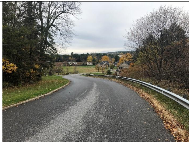
Photo 1: Top of drainage looking west towards Allen Brook
