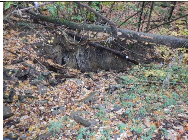
Photo 2: Large and active gully erosion from corner of parking lot to perennial stream channel
