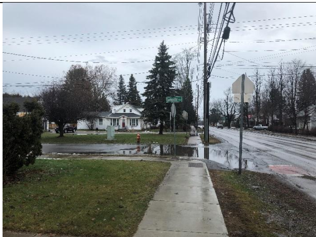
Photo 1: 3 Culvert under entrance to storage facility
