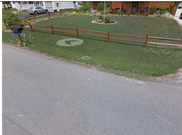
Photo 2: Existing dry well with grassed swale pre-treatment (Picture from Google Street View)
