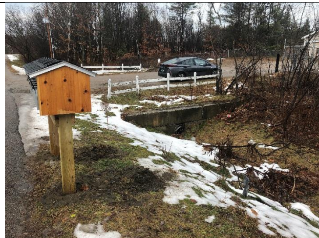
Photo 1: 3 Culvert under entrance to storage facility
