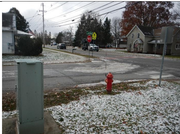
Photo 2: Runoff ponding on sidewalk along Checkerberry.
