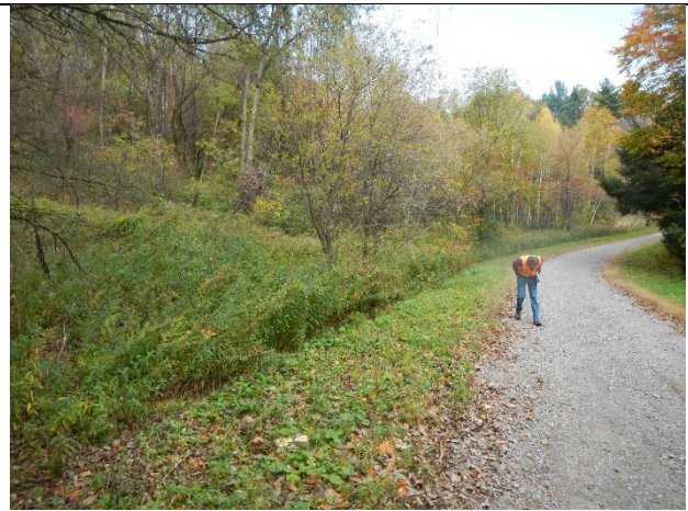
Photo 2: Rill erosion on road surface
