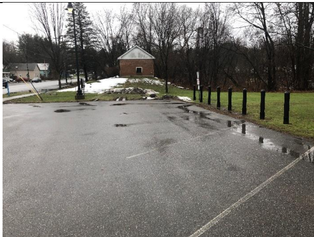
Photo 1: Runoff draining to southwest corner of parking area
