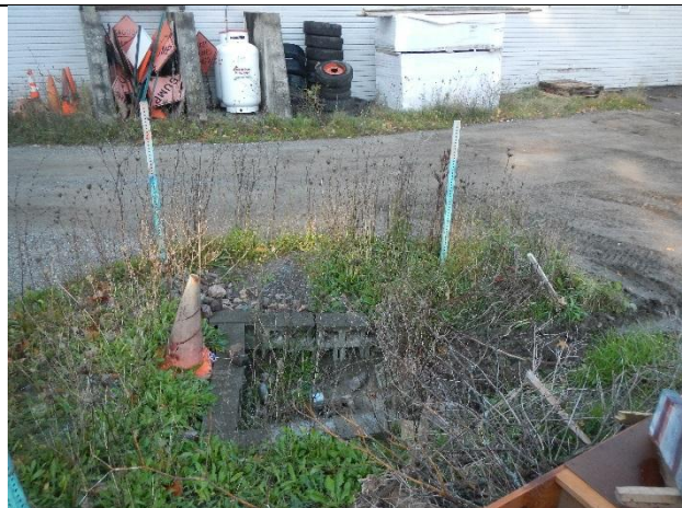
Photo 2: Deep catch basin with erosion
