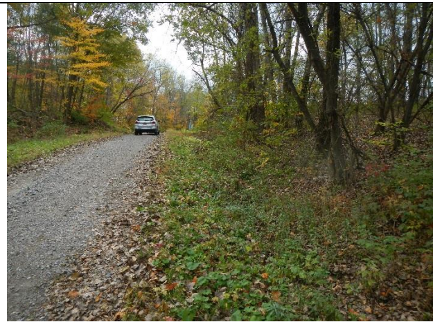
Photo 1: Minor gully erosion in ditch
