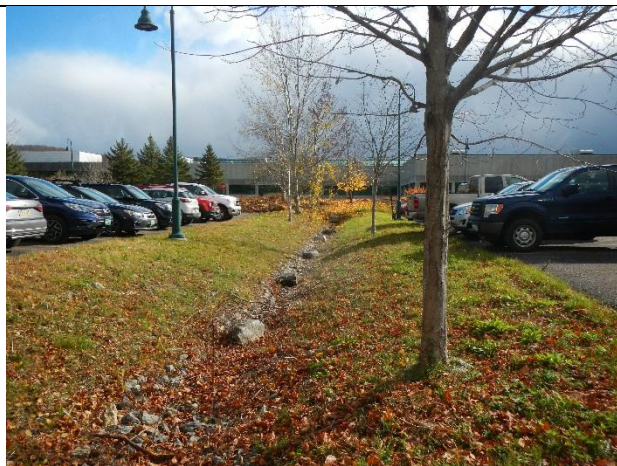
Photo 1: Stone lined swale between parking lots
