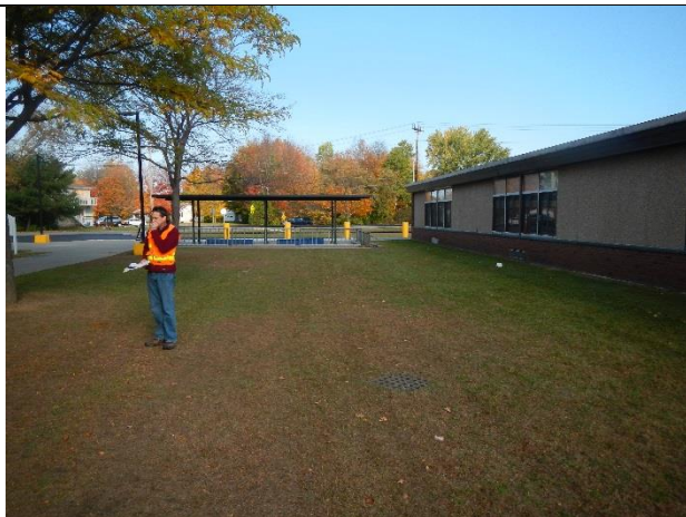
Photo 1: Catchbasin by main entrance (4a)
