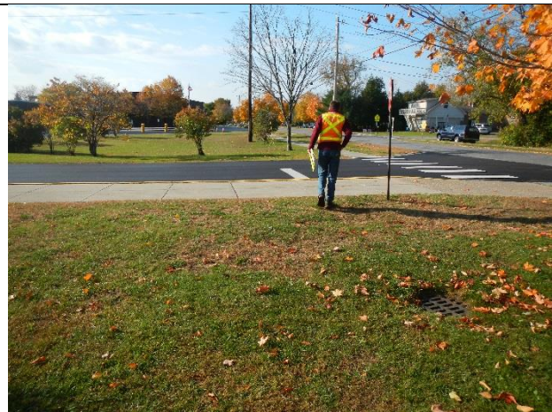
Photo 2: Catch basin draining south to large dry well and stream
