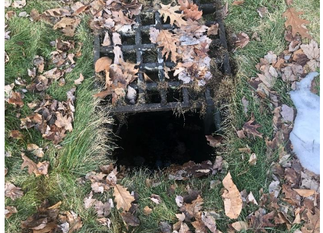
Photo 2: New 4-way shallow catch basin
