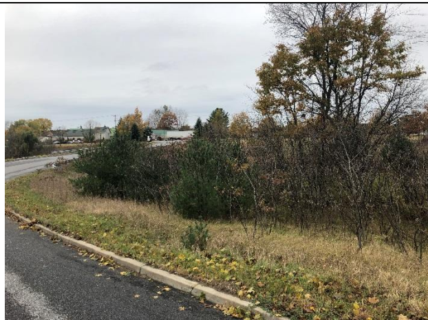
Photo 2: Location of proposed infiltration BMP – terrace located along the side of road above floodplain.
