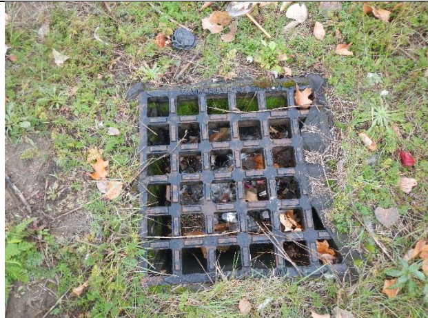
Photo 2: Fabric filter installed under catch basin grate
