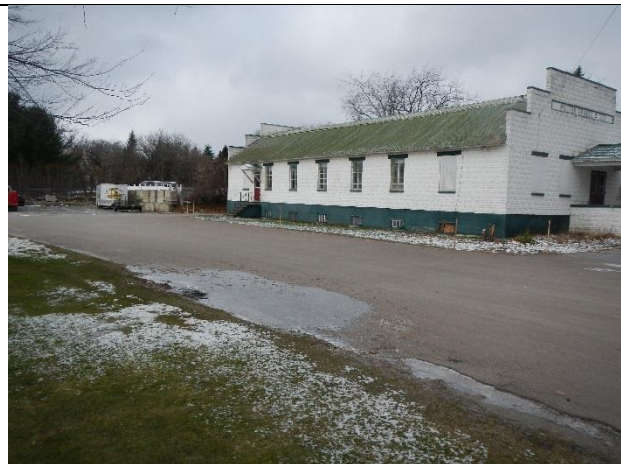
Photo 1: Grassed area with ponded water along southern edge of parking lot
