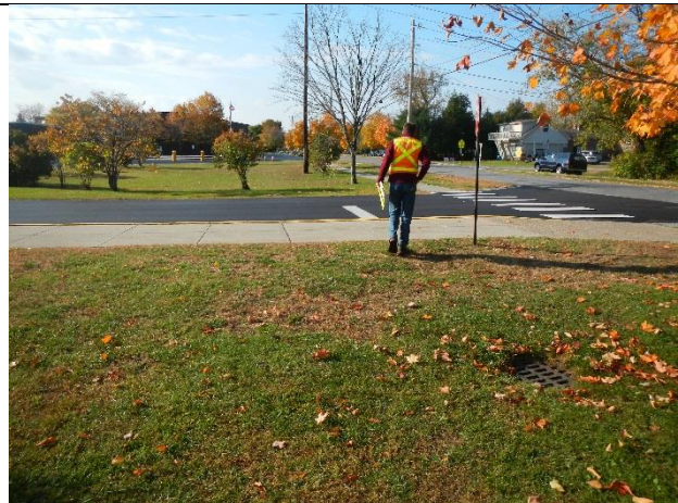
Photo 2: Catch basin connecting north parking areas to main drainage system
